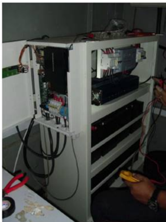
Solar power control box installation
