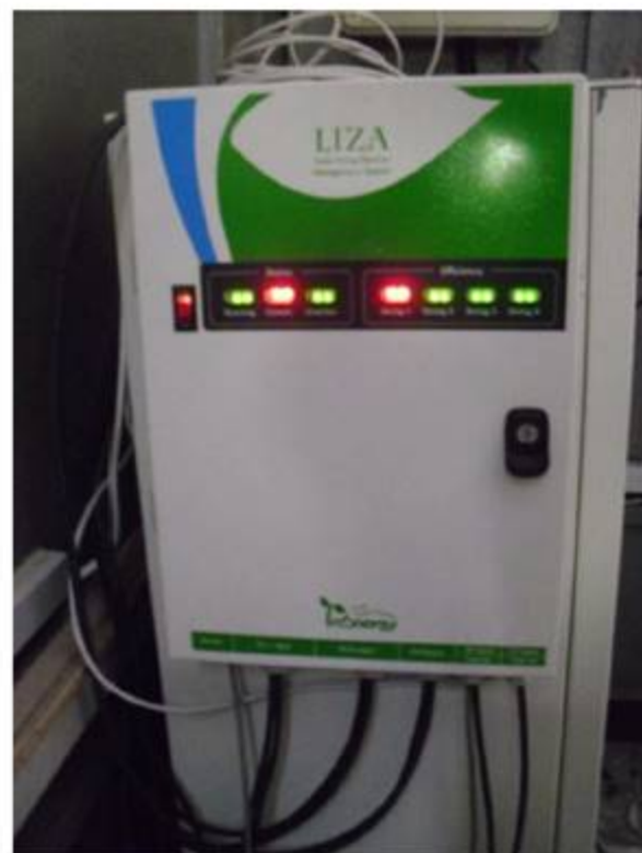
Solar power monitoring system installation
